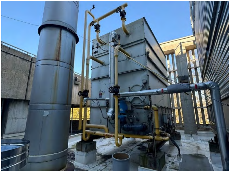
Abandoned ice system cooling tower
