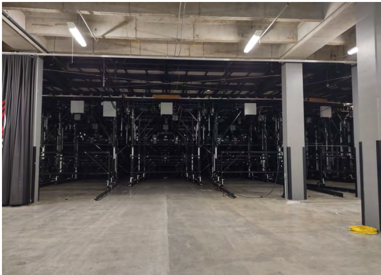
Undercarriage for new telescopic seating platforms
