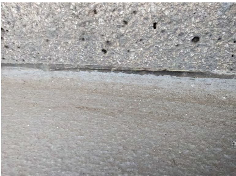
Suite level (Suite 41) plaza annex traffic coating upturn termination
