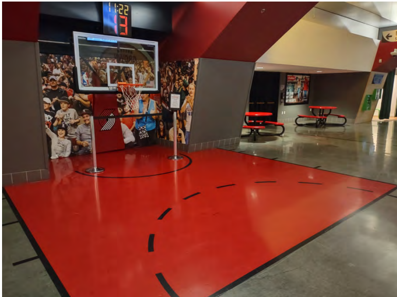
300 Level concourse architectural finishes are in good condition
