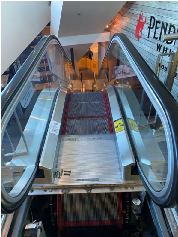
Proper protection from wall to unit
