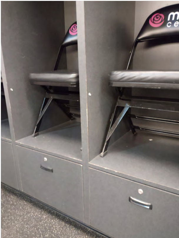
Lockers are original installation in Locker Rooms B and C, and show signs of wear and tear
