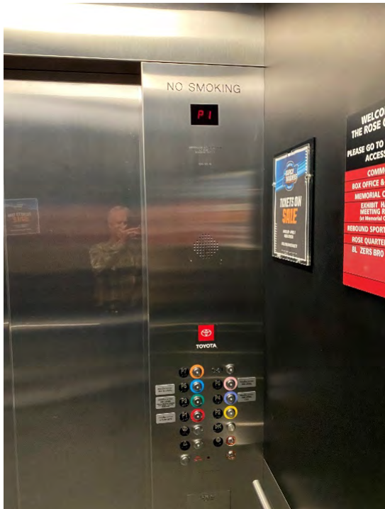
Typical elevator interiors for Elevators PE7 - PE10
