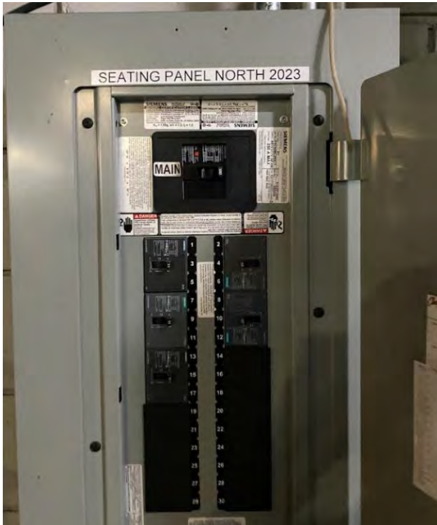
Typical retractable seating panel
