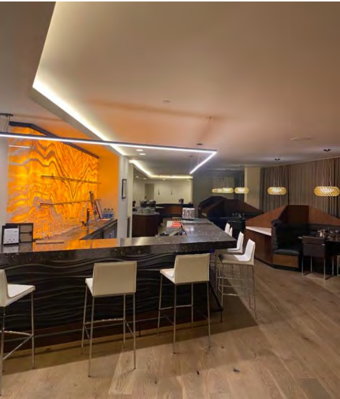
Club light fixtures
