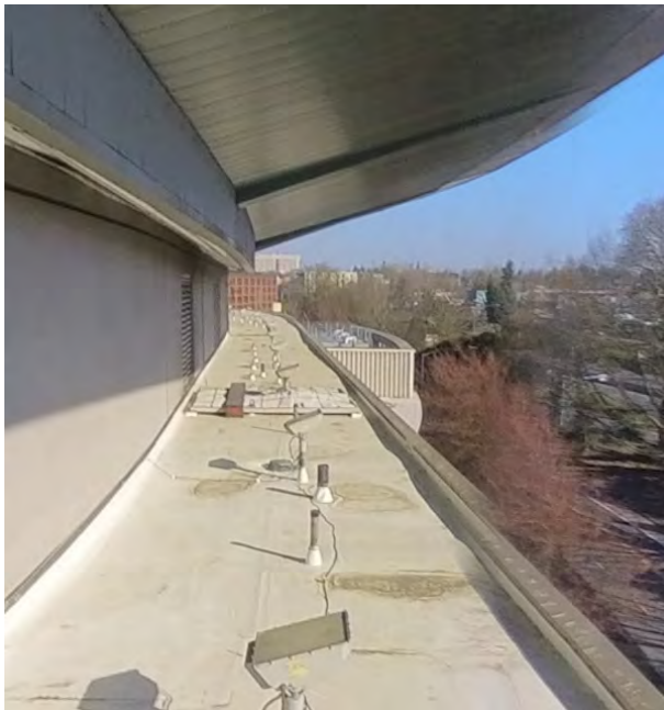
Vents and roof drains on level 7 intermediate roof
