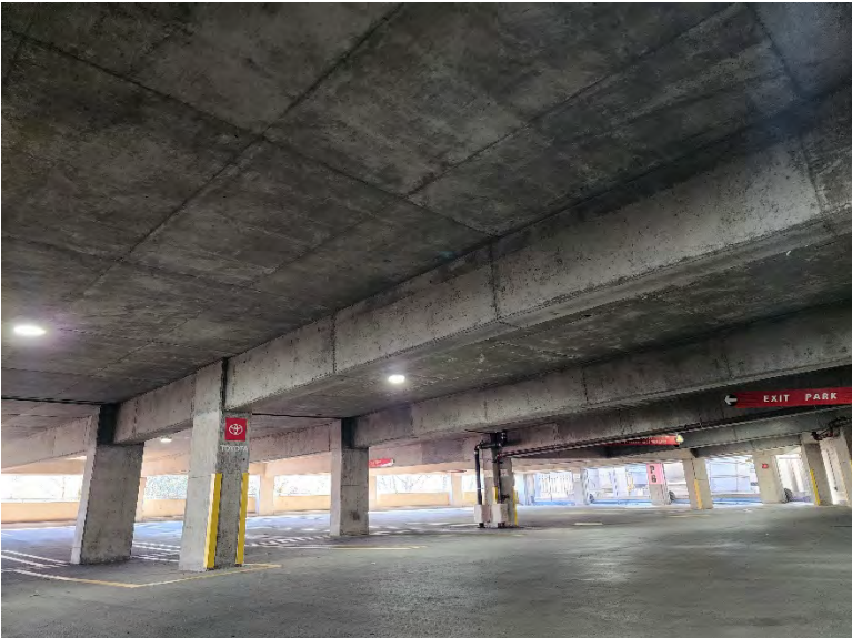
Level P6 post-tensioned slab spanning between beams spaced at approximately 20 feet on center
