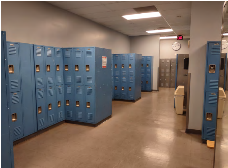
Staff locker room in fair to good condition
