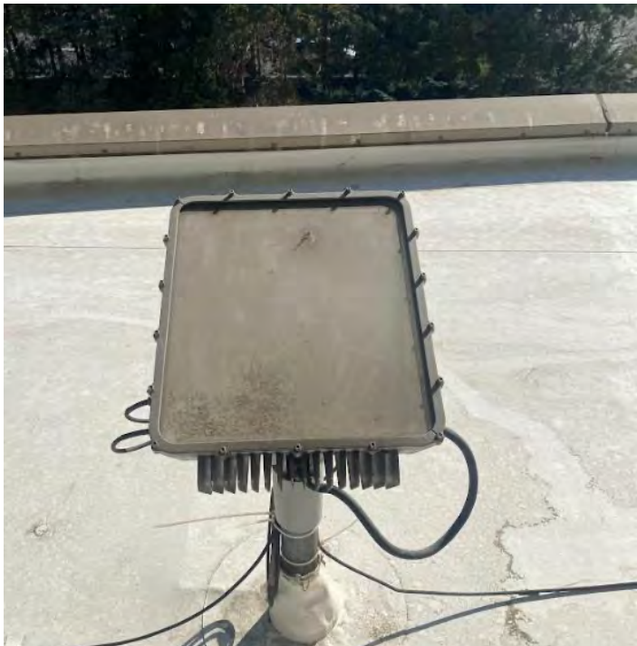
Low roof RGB fixture with dirty lens
