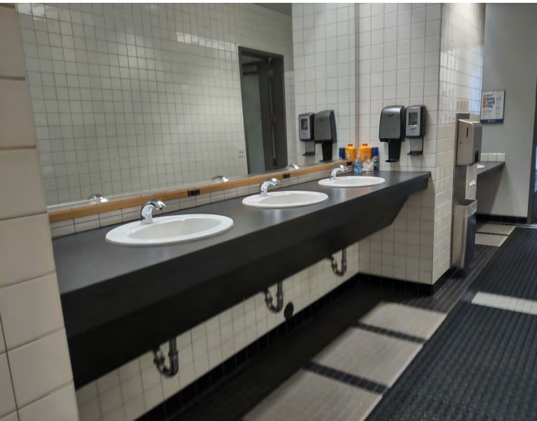
Team toilet rooms and showers are in good condition
