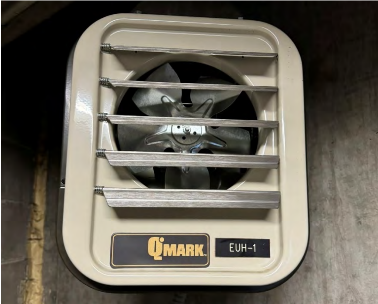
Electric unit heater
