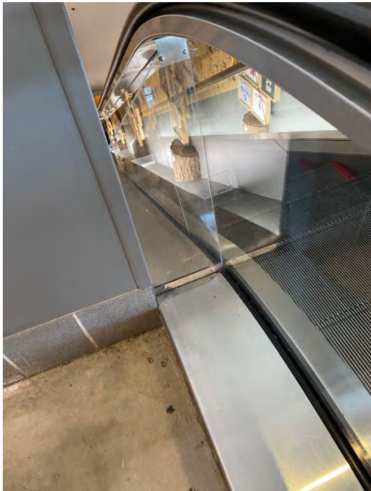
Proper protection from wall to unit
