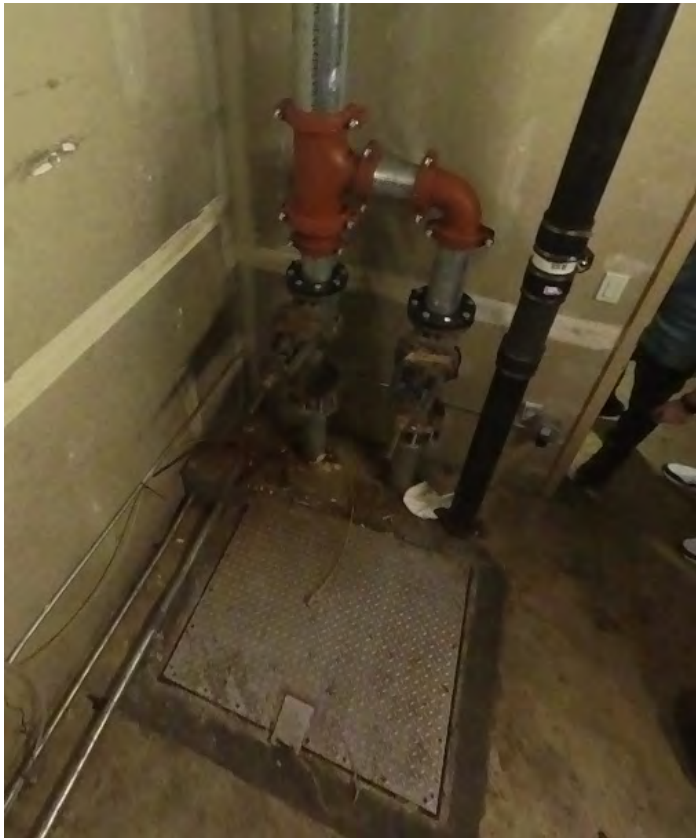
Ejector pit 1 on event level
