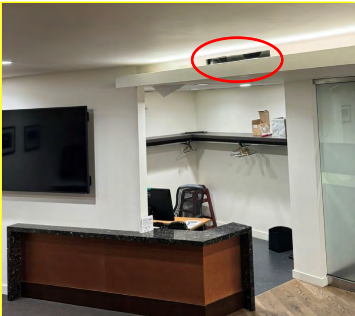
Missing diffuser
