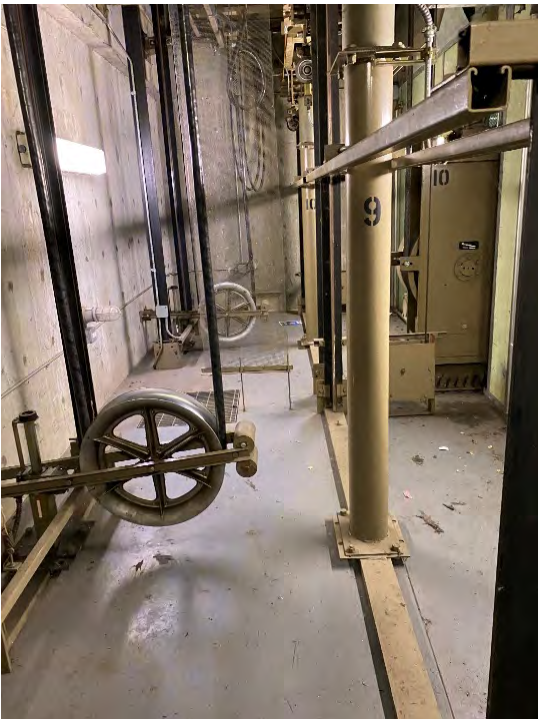
Pit equipment is clean and well serviced
