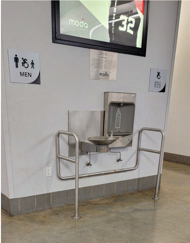
Polished concrete finish staining adjacent to walls
