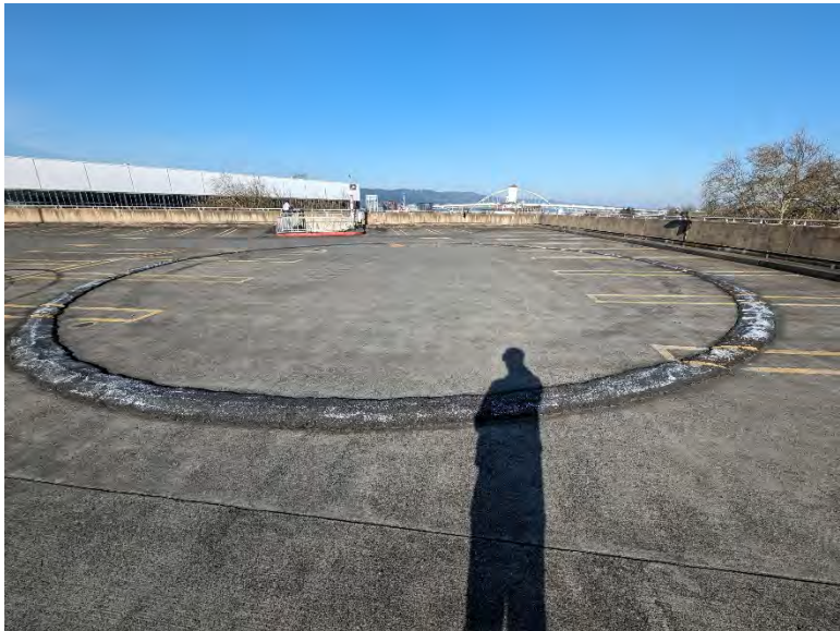
Level P7 helicopter pad
