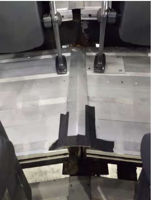
Aluminum closure plate at seating tread held in place with duct tape; this condition could become potential tripping hazard
