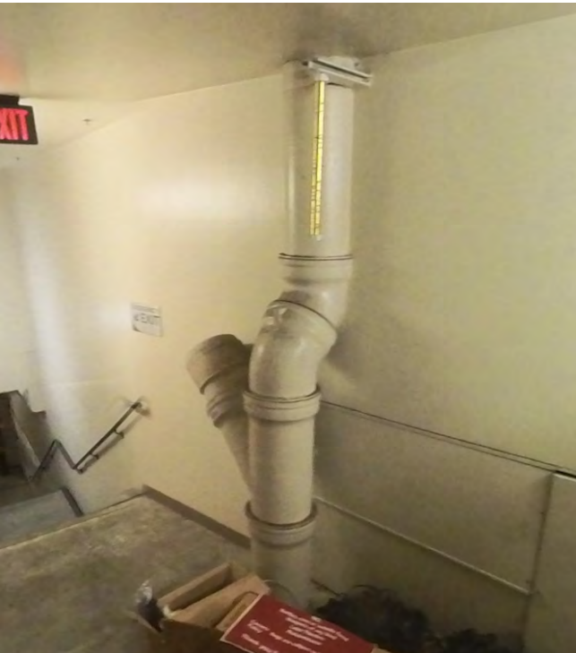
Storm water leader on southeast side of level 7
