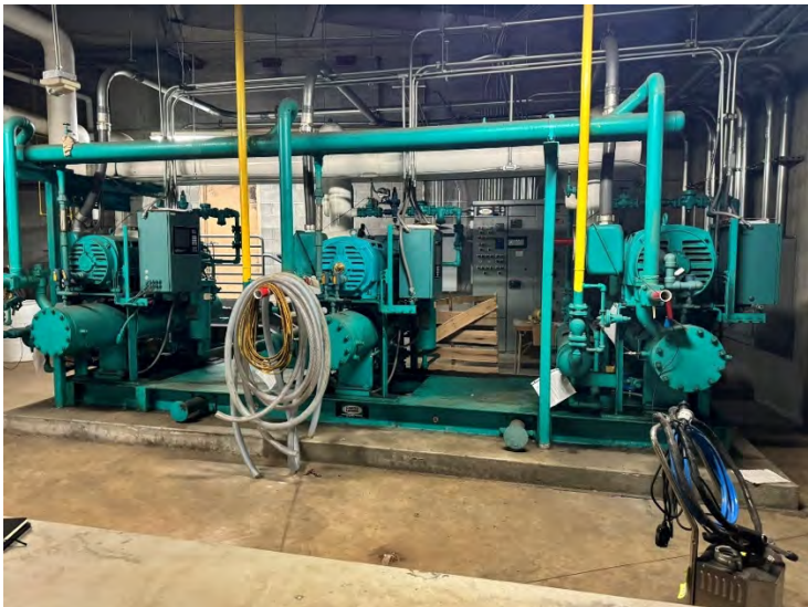
Abandoned ice chiller
