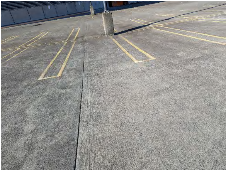
Level P7 floor slab construction joints
