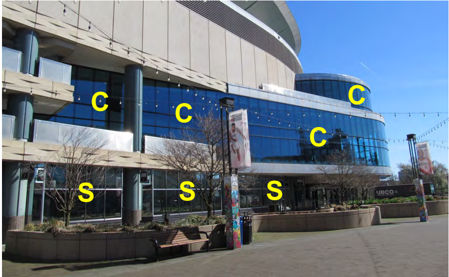
Areas of glass storefront (marked “S”, and curtainwall (marked “C”) along the west façade of the building
