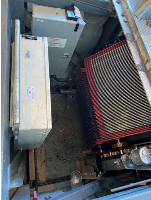
Escalator Esc. No. 2 with chains and tracks in good condition as well as the drive chain sprockets
