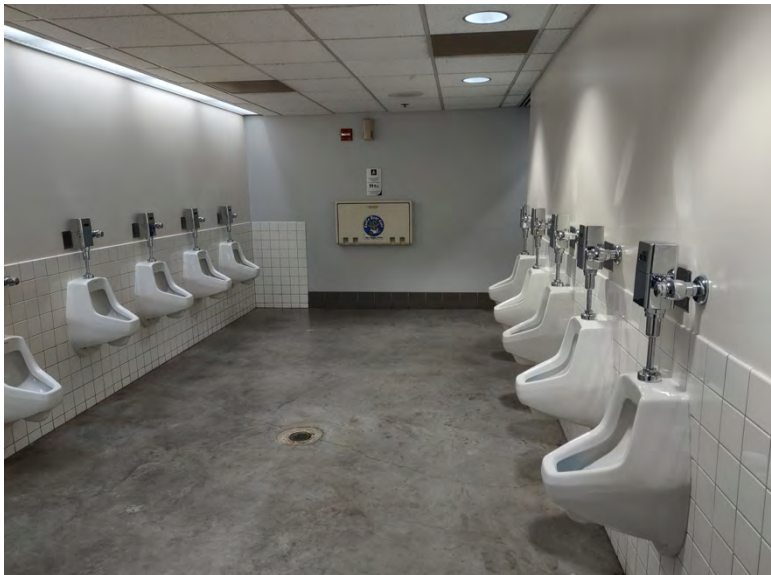
300 Level toilet rooms have original finishes
