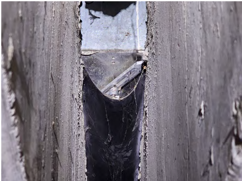
Level P2 underside of expansion joint
