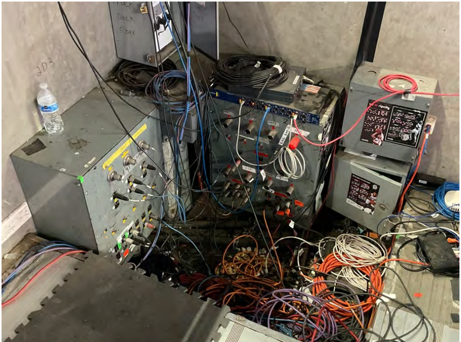
Main camera platform broadcast cable panels
