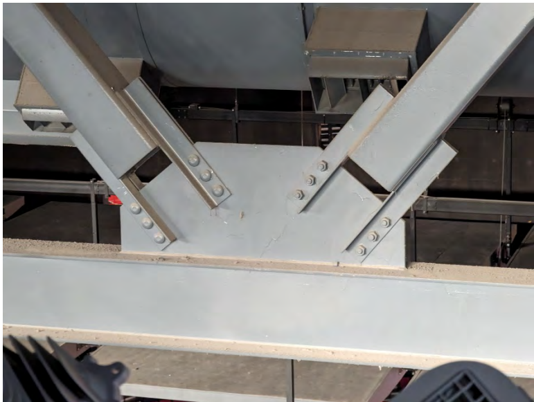
Catwalk level steel framing bolt connection
