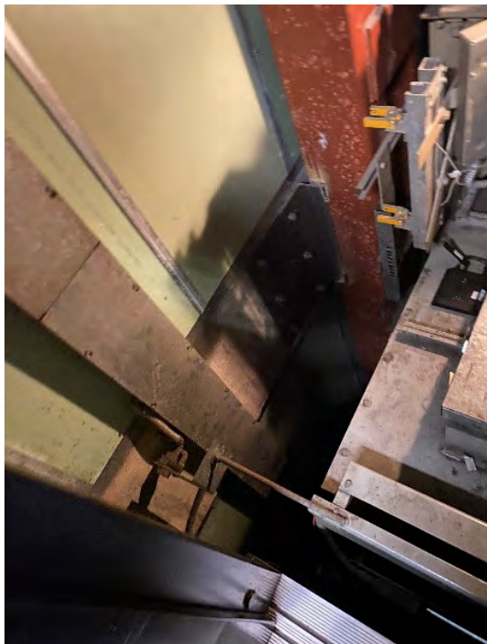
The existing opening between the car and the shaft wall is 26" x 28" wide
