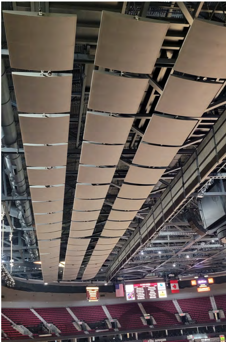
A unique feature to the Moda Center known as the "acoustical cloud"
