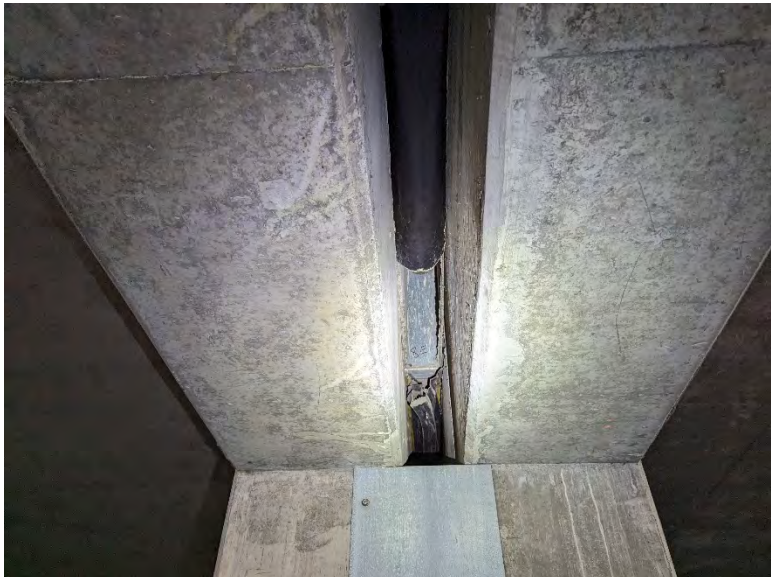
Level P5 underside of expansion joint
