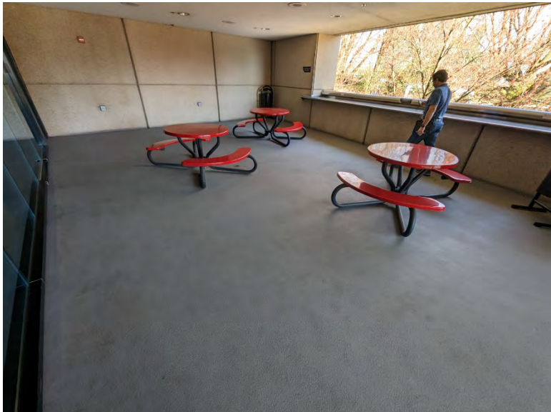
Suite level (Suite 41) plaza annex traffic coating
