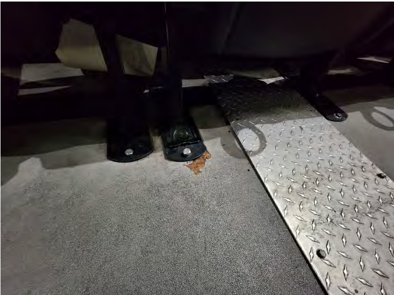
Seating bowl (Section 326) with installed metal protection plate over joint sealant
