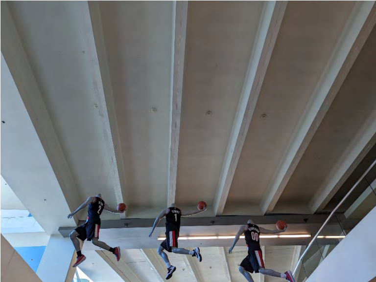
Upper concourse (Section 321) concrete pan joist soffit
