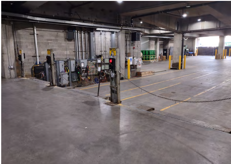
The loading dock is in fair to good condition, showing signs of normal wear and tear
